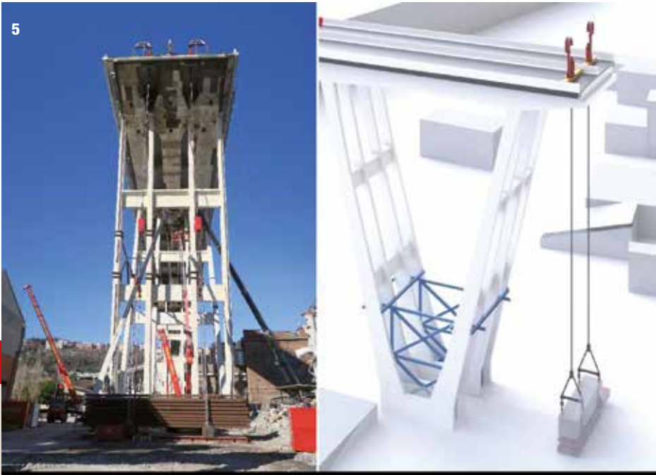
4. Main strand jacking operations 5. Counterbalance system 6. Fagioli Cantilever Beam System
