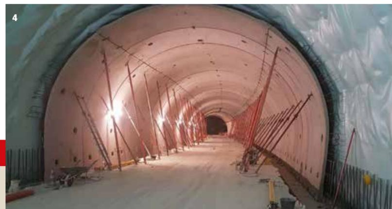
3. A1 motorway, South Florence, Antella tunnel: double slab retaining walls
